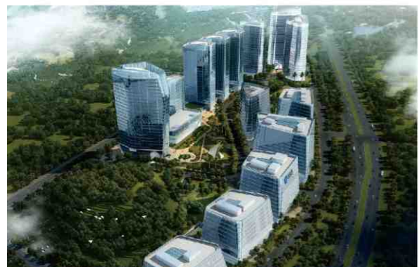
Leadshine Headquarters in Shenzhen
